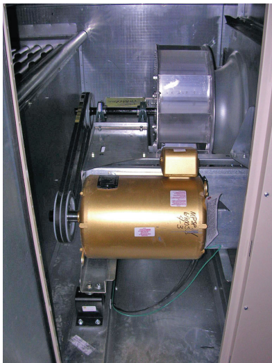
Figure 6: Fan Section (MPS 015–050)
